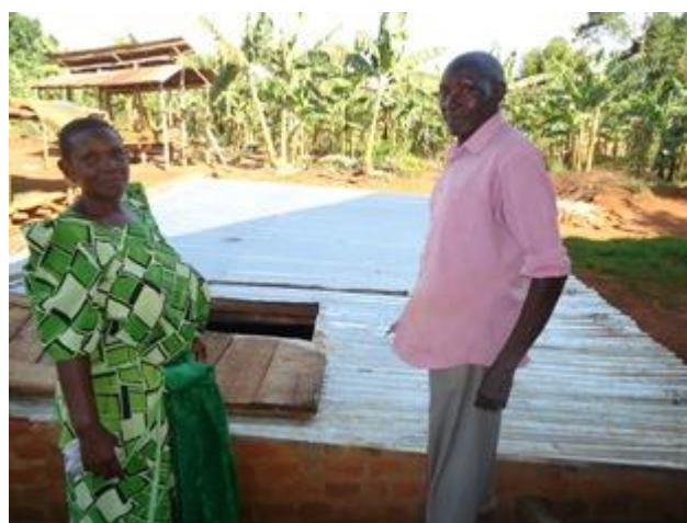
Rain water harvesting tank at the Ddakis
